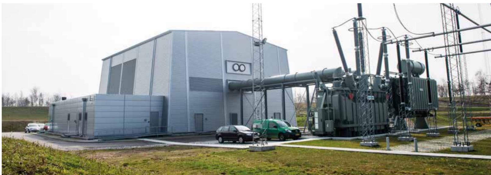
Figure 4 – Example of typical Synchronous Compensator – for indicative purposes only
